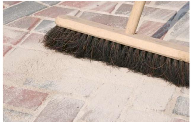
Jointing sand is simply applied by brushing into place with a soft broom. Joints should be filled at least 25-30mm with approved sand. This typically applies to refurbishment of existing pavements. New construction should be filled 100% joint depth.
