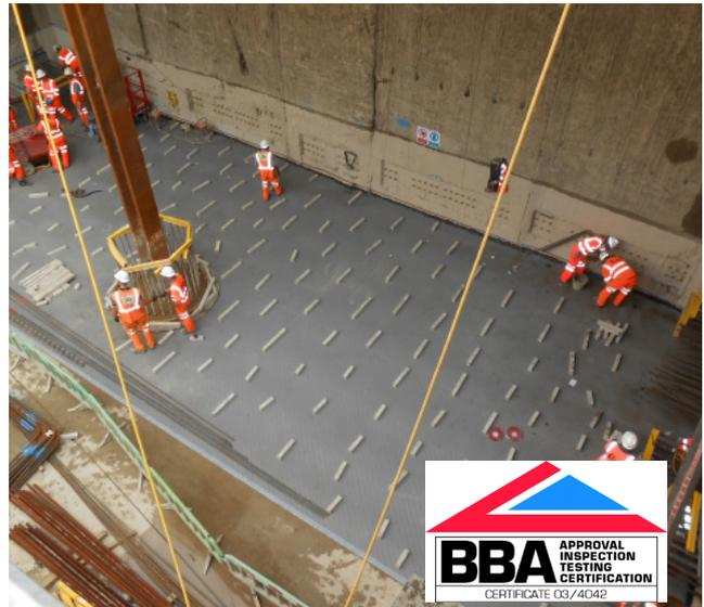
Where ground gas protection is required Proofex Engage, in conjunction with Supercast Watertight Concrete, has been independently assessed as providing a score of up to 4.5 points sufficient for all building types constructed in ground with a Characteristic Situation 3 hazard potential.
