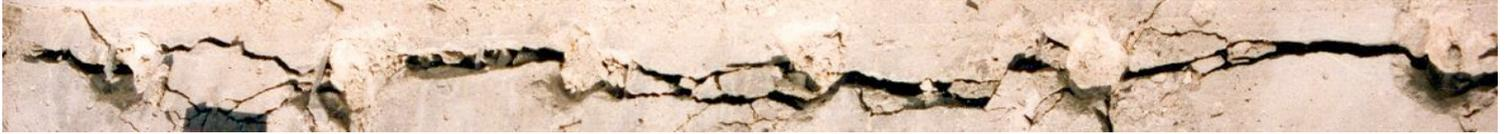
**Empty holes "repel" cracks.** A row of empty holes sets the breaking boundary.
