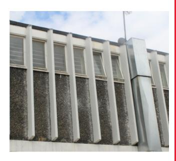
of Dekguard Elastic achieving a wet film thickness not less than 400 microns per coat. The product application shall be in accordance with the manufacturer's written instructions to a correctly prepared substrate.
